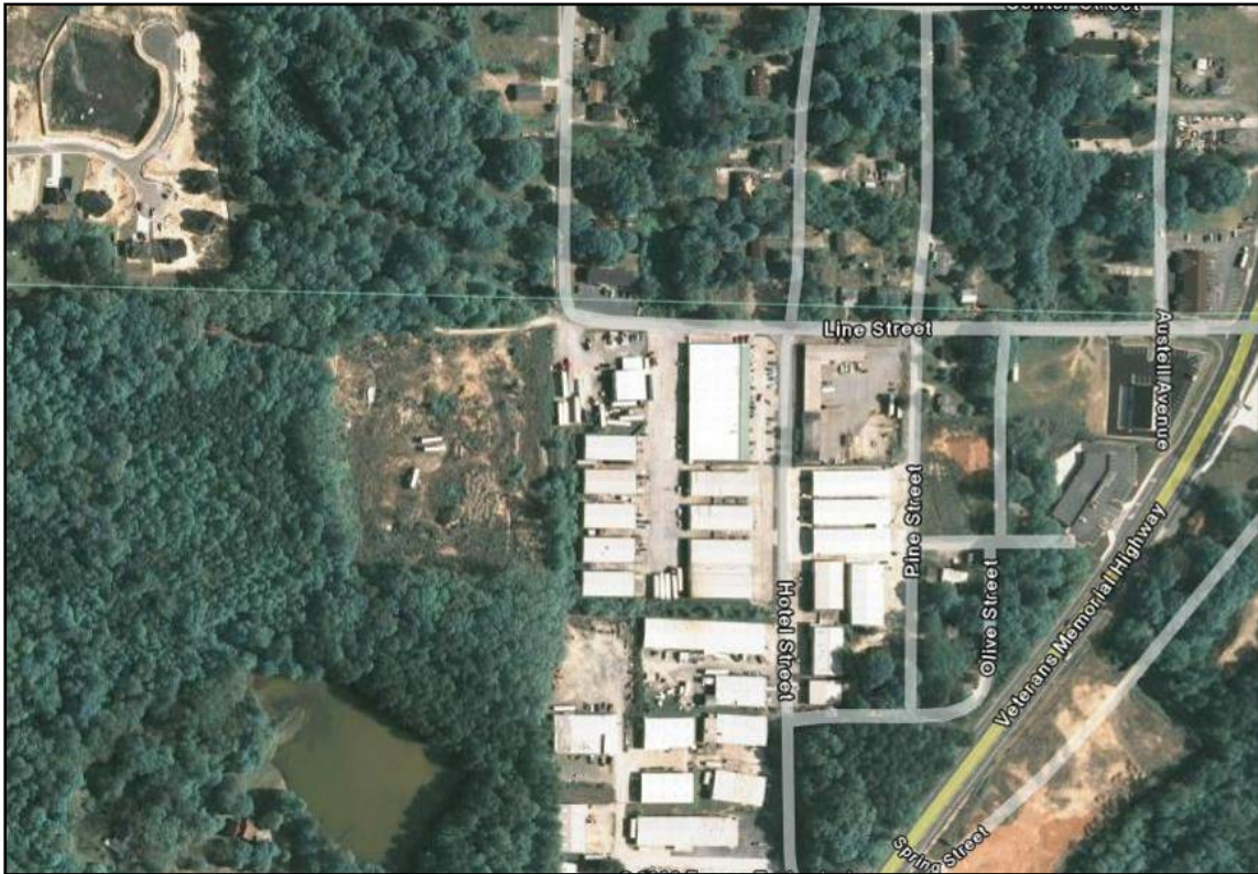
Figure 36 – Freight facility near US 78
